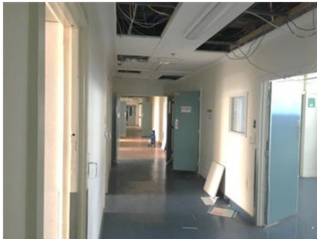
Level 8 – Main Corridor (Photo Jan 2018)
